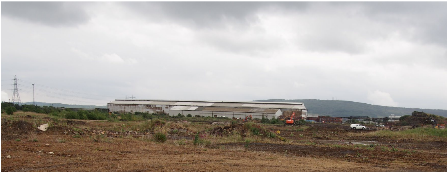
Plate 3: Torpedo Ladle Workshop from the north
